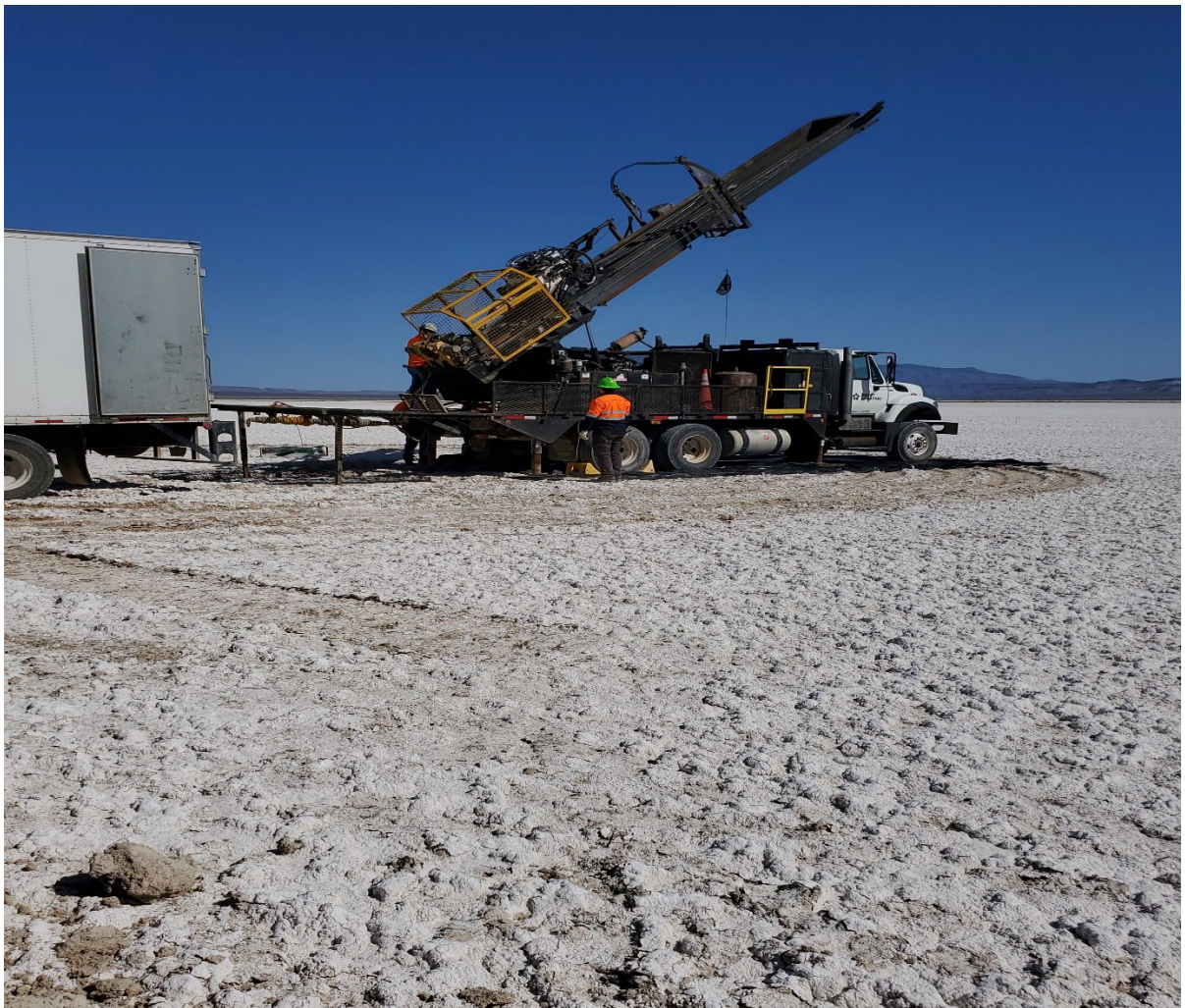
Figure 4-18 Drillers Setting up LS™600 Sonic Drill Rig on Drill Pad.
